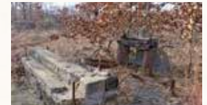
Concrete oil pumpjack stands from 1911-1945
